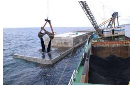
Filling a caisson with slag
