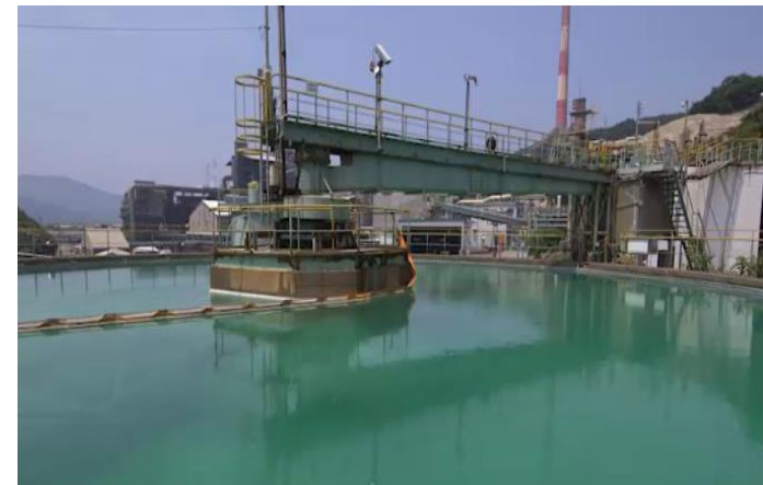
Waste water treatment plant
